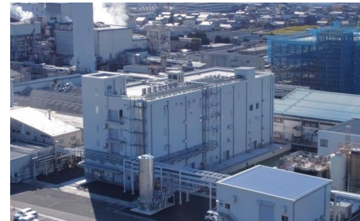
Appearance of new equipment for culture and purification at Tsuruga Biochemicals Plant
