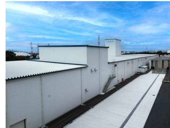
Appearance of new production facility
