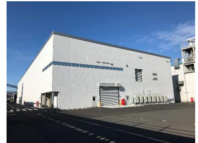
Tsuruga Films Plant Coater Building
