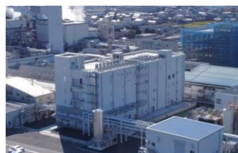
Appearance of new equipment for culture and purification at Tsusuga Biochemicals Plant
