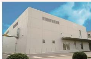
Otsu Pharmaceuticals Plant
