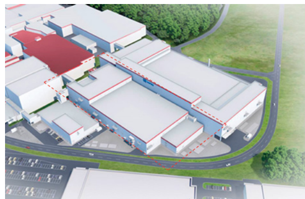
Integrated production plant for dialyzers
