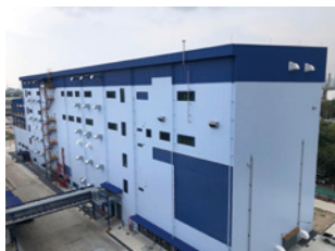
Completion of a nylon yarn production plant for TIAF's airbags on the grounds of IPI
