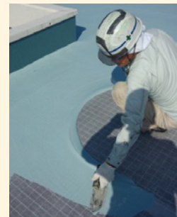
Applying waterproof material coating to ventilation buffer sheets
