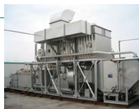
VOC recovery equipment
