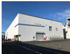
Coating equipment for mold releasing film for MLCC Tsuruga Films Plant Coater Building
